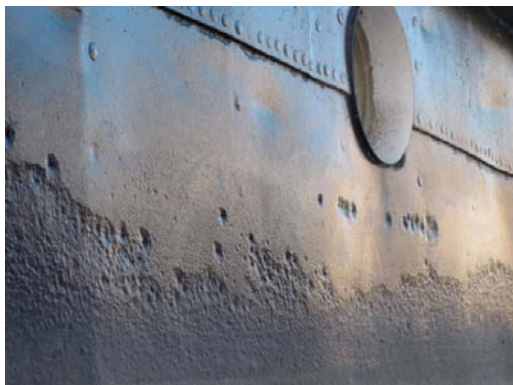
Pitting on topsides
